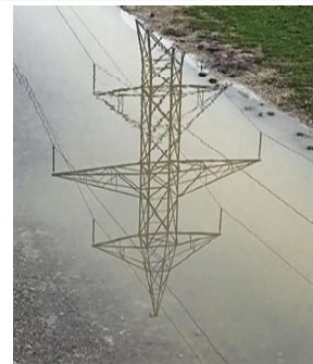
Transmission Tower Reflecting in Puddle
